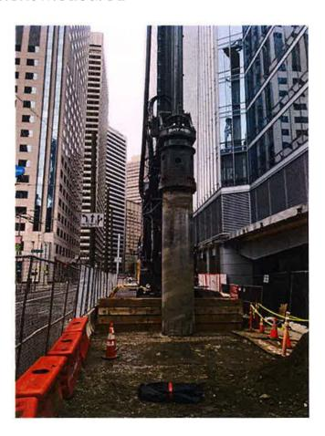
The foundation upgrade has been likened to putting a bumper jack next to a flat tire. It relies on drilling and jacking 52 concrete piles—socketed more than 30 ft into the bedrock that starts 220 ft below grade—under the tower's north and west sidewalks.
