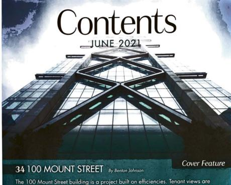
maximized with an offset core and 20-foot column-free cantilevered zones. The offset core is balanced by an innovative composite mega-bracing system.
